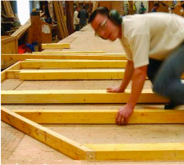
Constructing a timber frame in a factory
